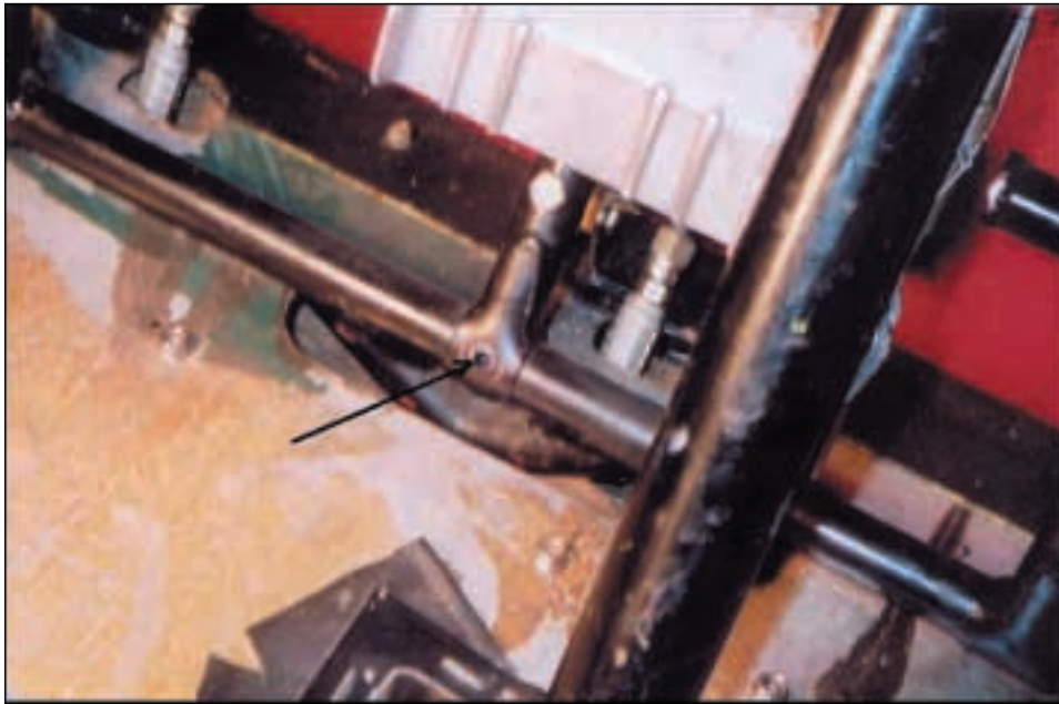
A view of the pilot's RH pedal showing the elongated hole with the bolt removed
