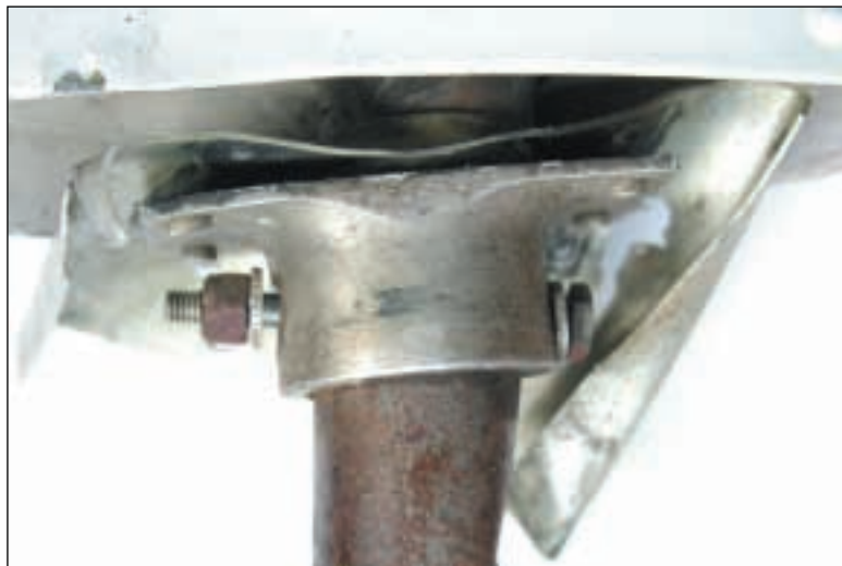
Spar /fuselage attachment bolt, nut and washer. Note long bolt and space between washer and housing.
