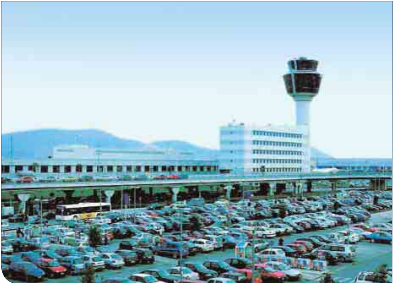
© Athens International Airport
