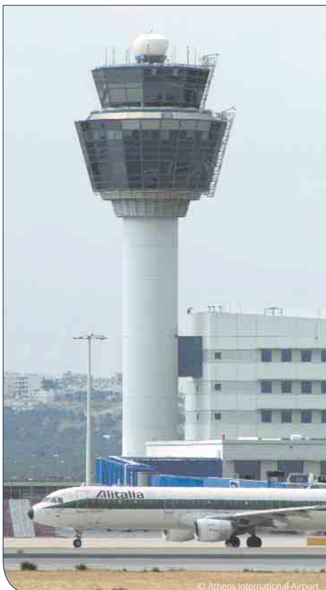
© Athens International Airport
