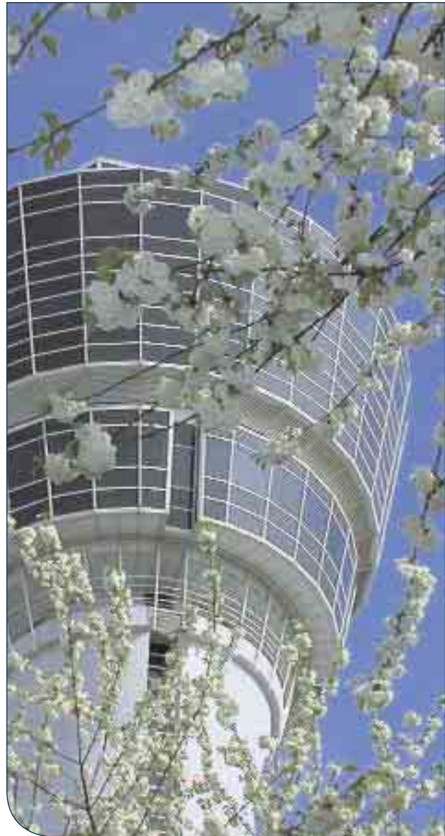
© Athens International Airport
